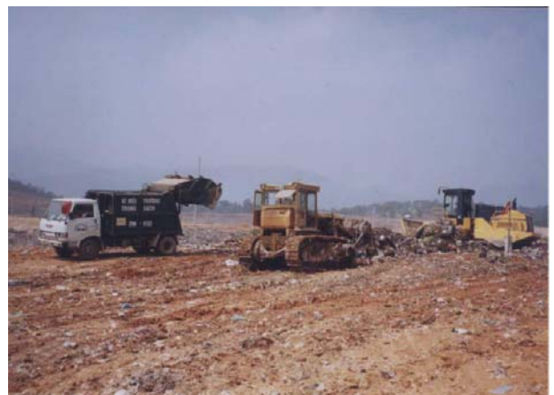
The Hanoi landfill site in operation
