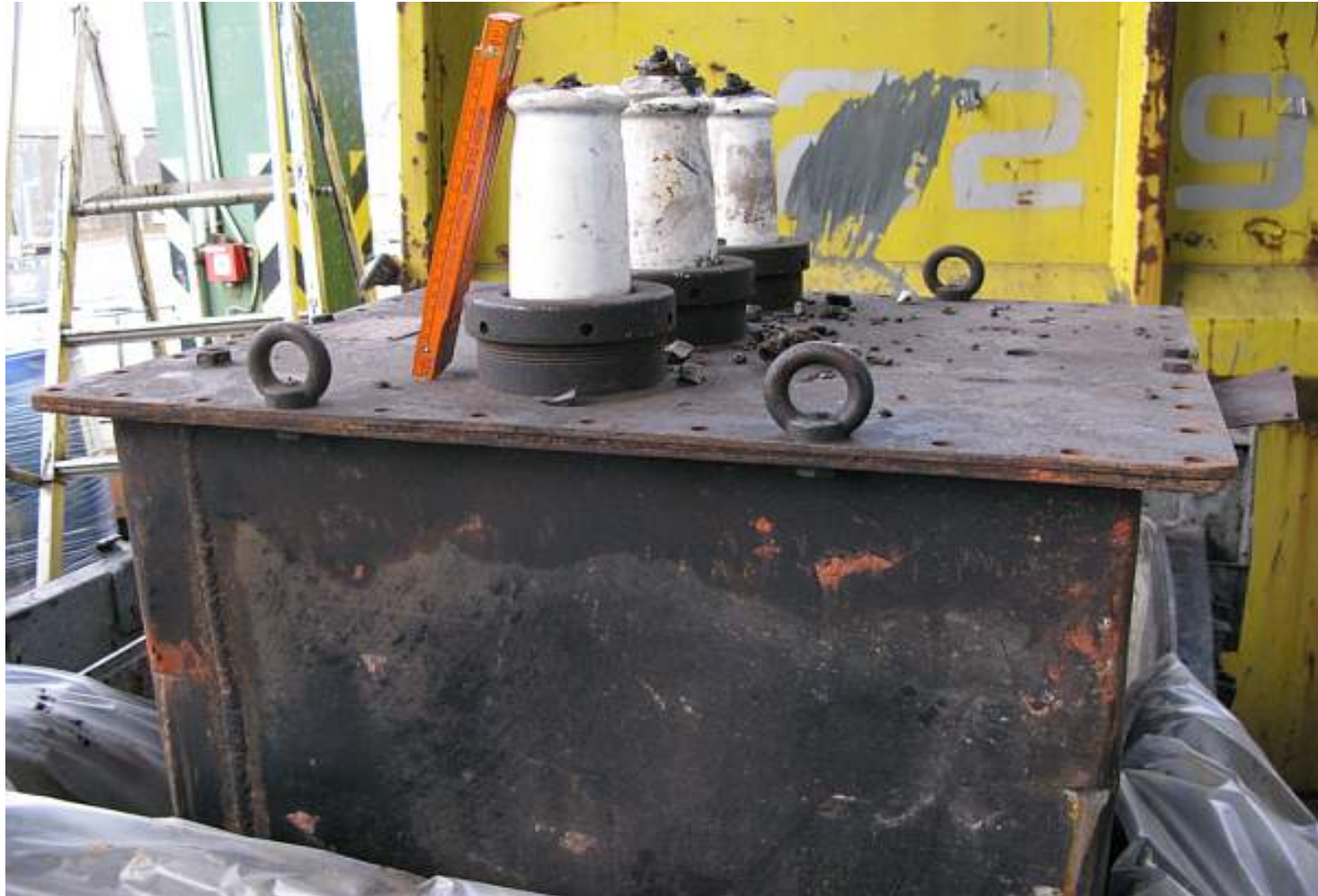
Capacitor filled with PCBs at idr-eg's decontamination site for hazardous waste, Düsseldorf
